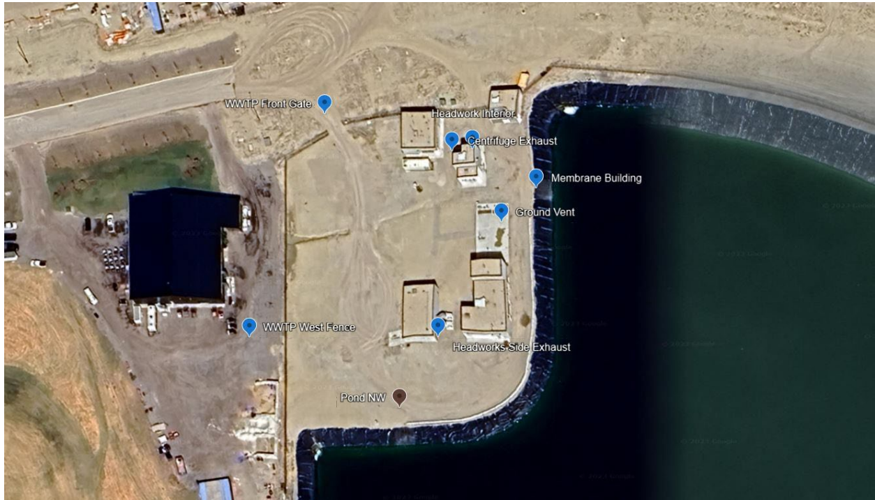
Figure 5: Aerial view of Harmony Wastewater Treatment Facility, with several points of interest indicated.
